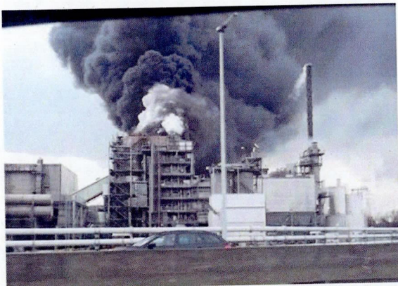
Figure 1: Antwerp facility explosion in 2018
